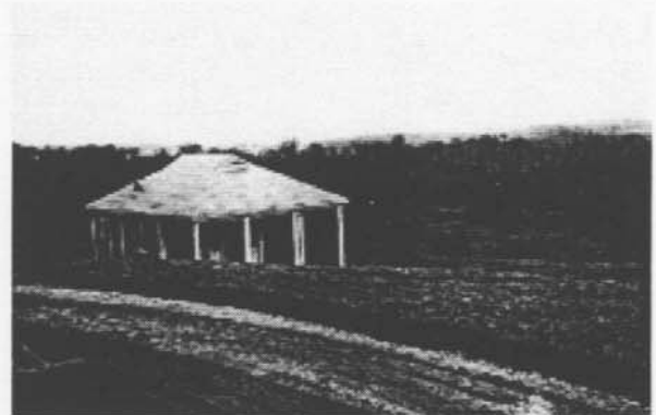
Figure 17: View northwest to 1927 pavilion, c.1950 (Source: OPRHP)
